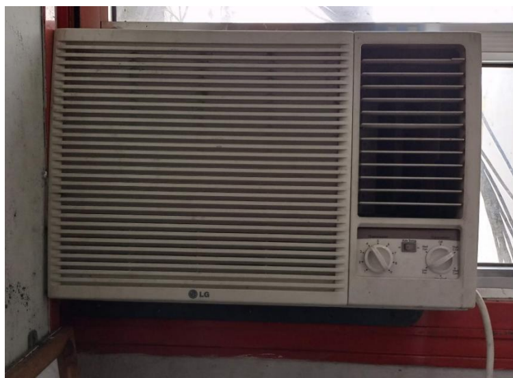
Figure 7: Window air conditioner
