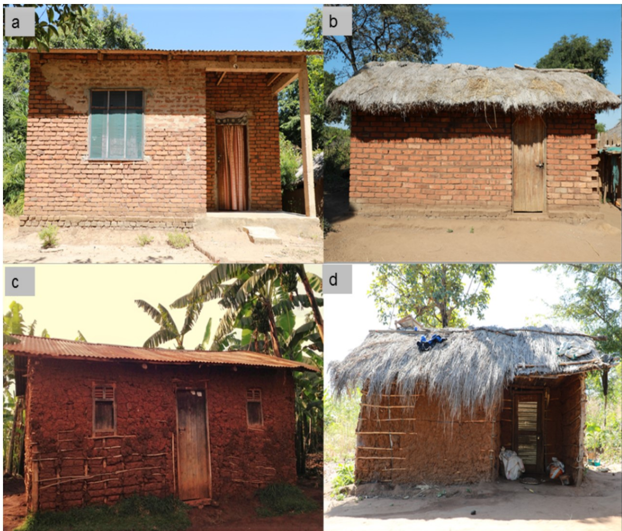
Figure 6: Common house type in the study sites: a) brick walls with metal roof, b) brick walls with thatched roof, c) mud walls with metal roof, d) mud walls with thatched roof
