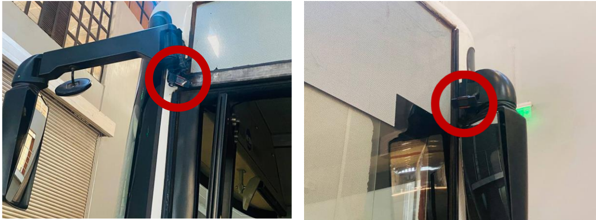
Figure 23: Installation of the right and left-hand side cameras
